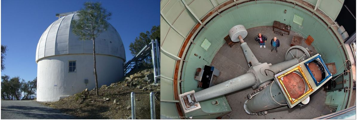
Fig. 3. LEFT: Exterior of the Astrograph dome is scheduled to be refurbished this year. RIGHT: Astrograph telescope mount and dual refractor telescopes with wood lens covers at the top. Our proposed plan is to make use of the dome and mount, and remove the dual telescopes for storage.
